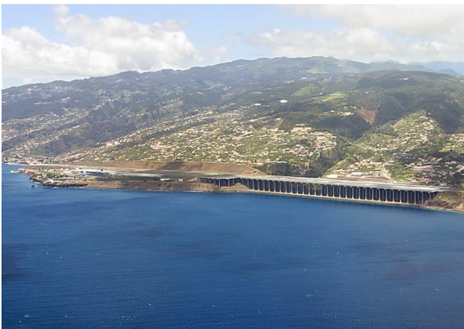
The interesting runway construction of Madeira Airport Photo by Peter Fagerström
