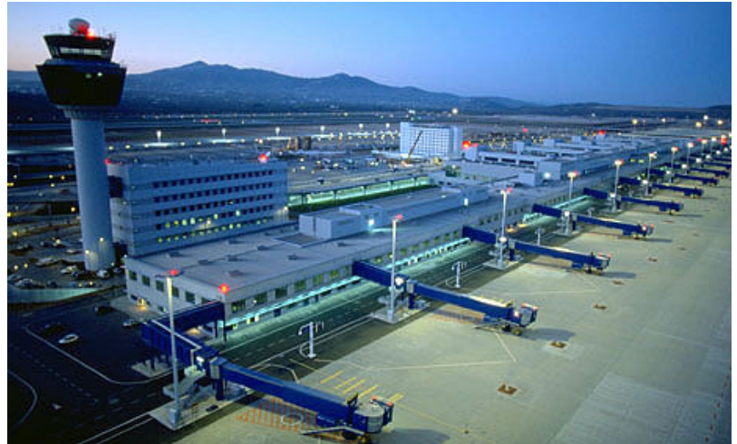
Photo 1: The gates and Terminal building. Courtesy of www.greece-athens.com
